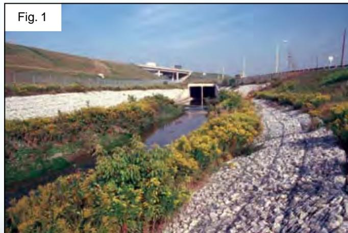
Maccaferri double twisted hexagonal wire mesh is manufactured from heavily galvanized steel wire, with a tough PVC coating for additional protection.
